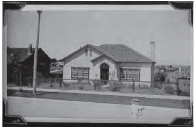
Exterior of the authors home in Hassetts Estate Photograph taken by the authors father
